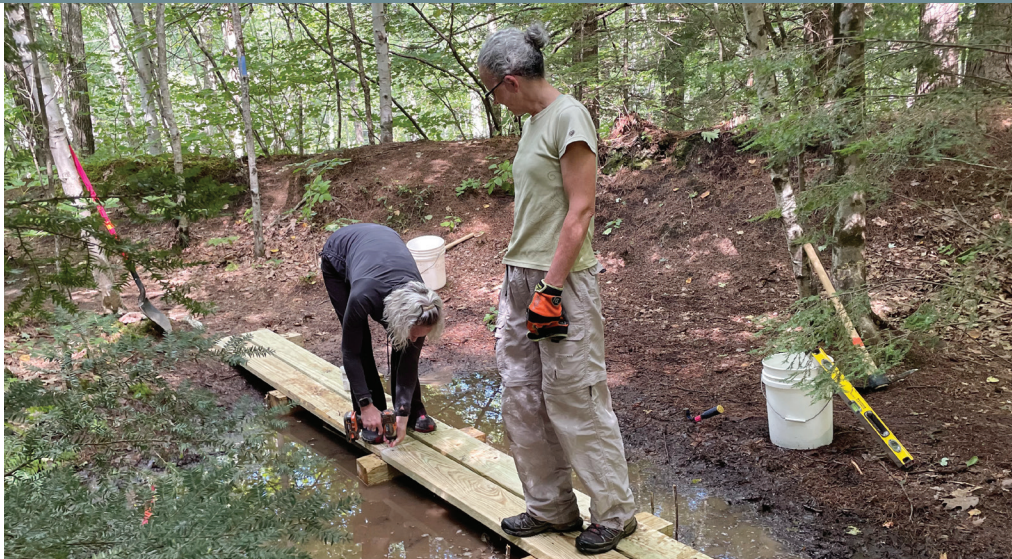
Bog bridge installation workday at Keay Brook
