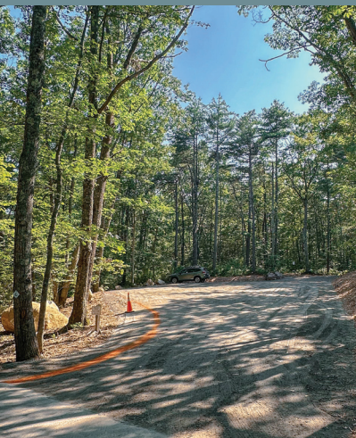
New and improved Kenyon Hill Preserve parking area
